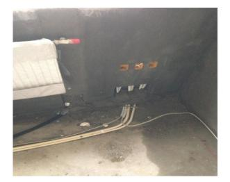
The picture illustrates the installation of radiator. As we can see that the radiator is placed under the window and the pips are covered that the water is not getting cold tell it reaches the radiator, we can see 2 pips which connected to the radiator the hot water comes from one side and go out again from another side.
