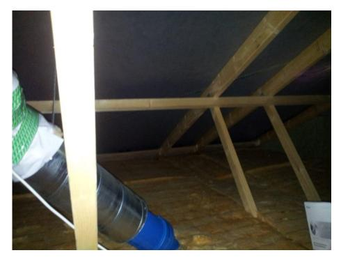
We climbed up to the attic we saw inside of the attic above the ceiling, here we can see the trusses and rafters which carry the load of the roof, mineral wool is placed on top of the ceiling.
