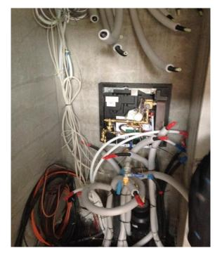
The shaft is placed in the entrance of the ground floor where all installations are connected to the shaft and the pips are divided to different parts of the house, the shaft base is in the ground floor and there is only a small hole in the first floor partition where the pips for radiators and wire for electricity comes out.
