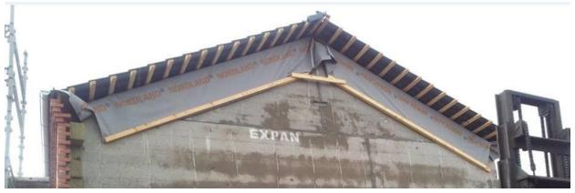
The pictures shows the external part of the roof where we can see the slops, which has created a attic the damp proof membrane is a diffusion open. The membrane is stretched and tight to two sides of gables to to protected it from blowing of the wind and water d it allows moisture go out.
