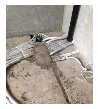
Her we can see that for the first floor we don't have shaft only a hole where the pips come and then the hole is covered by mortar. When the installation is finished all the installation cables and pipes will be hidden under the flooring.
